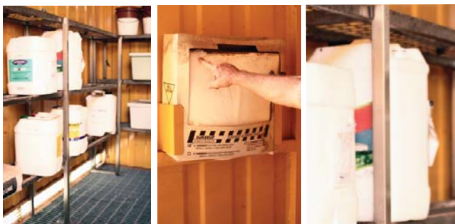
Bunded floor through grate with ground level cross airflow and also absorbent material.
